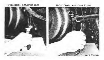
Figure 38—Tronsmission Mounting Nuts and Chain Adjusting Screw
