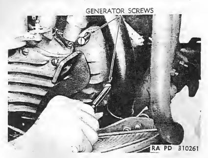
Figure 58-Removing Generator End Mounting Screws
